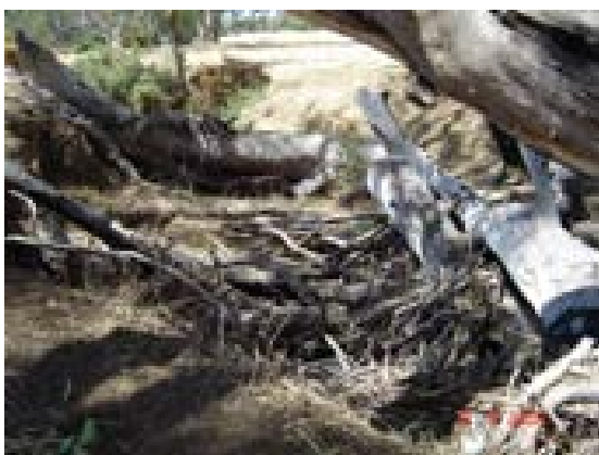
■ Figure 4-1 Woody debris jamb on G1/2 upstream of Nowhere creek road
