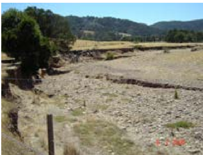
■ Figure 7-4 Bed & bank erosion as a result of stream straightening and diversion
