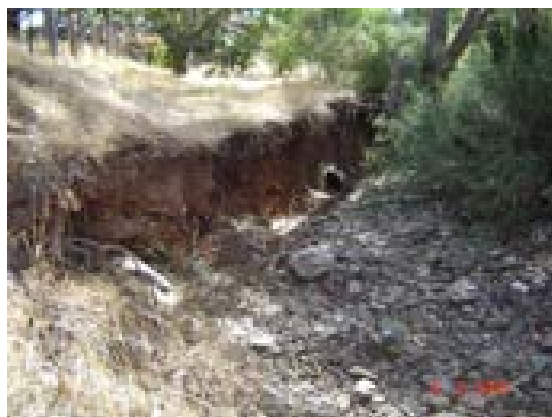
■ Figure 5-3 bank erosion due to historic stream straightening of Glenpatrick Creek
