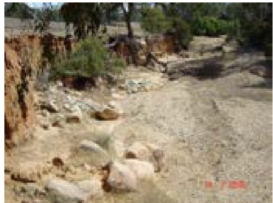
■ Figure 4-2 Previous rock treatment to try and prevent bank erosion
