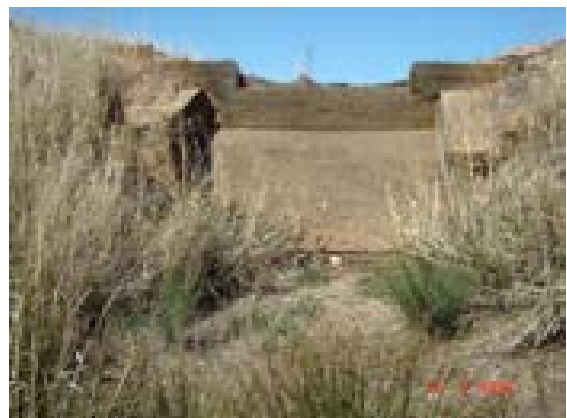
■ Figure 6-4 Existing concrete drop structure on W5/3/1/2
