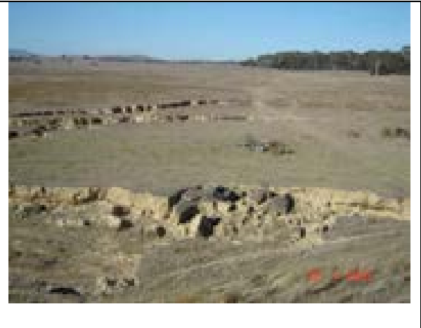
Figure 7.3 – Tunnelling and subsurface flows are contributing to erosion
