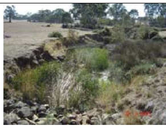
Figure 4.3 – Big Hill Road crossing requires appropriate stabilisation to prevent further erosion
