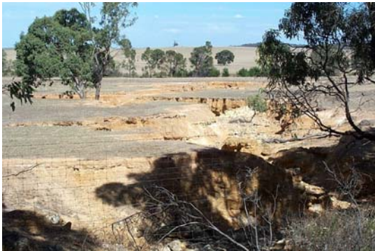
Figure 15: Eroding tributary of Surridge Creek
