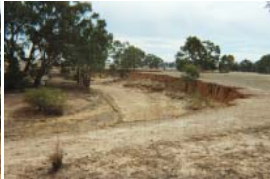
Figure 12: Enlarged channel & uncontrolled stock access to Seven Mile Creek, Reach 4
