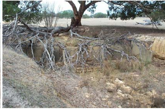
Figure 3: Drop structure at upstream end of Reach 2
