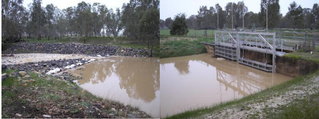
Figure 3-15. Huddleston's Weir (left) and the adjacent gates on the Wimmera Inlet Channel (right)
