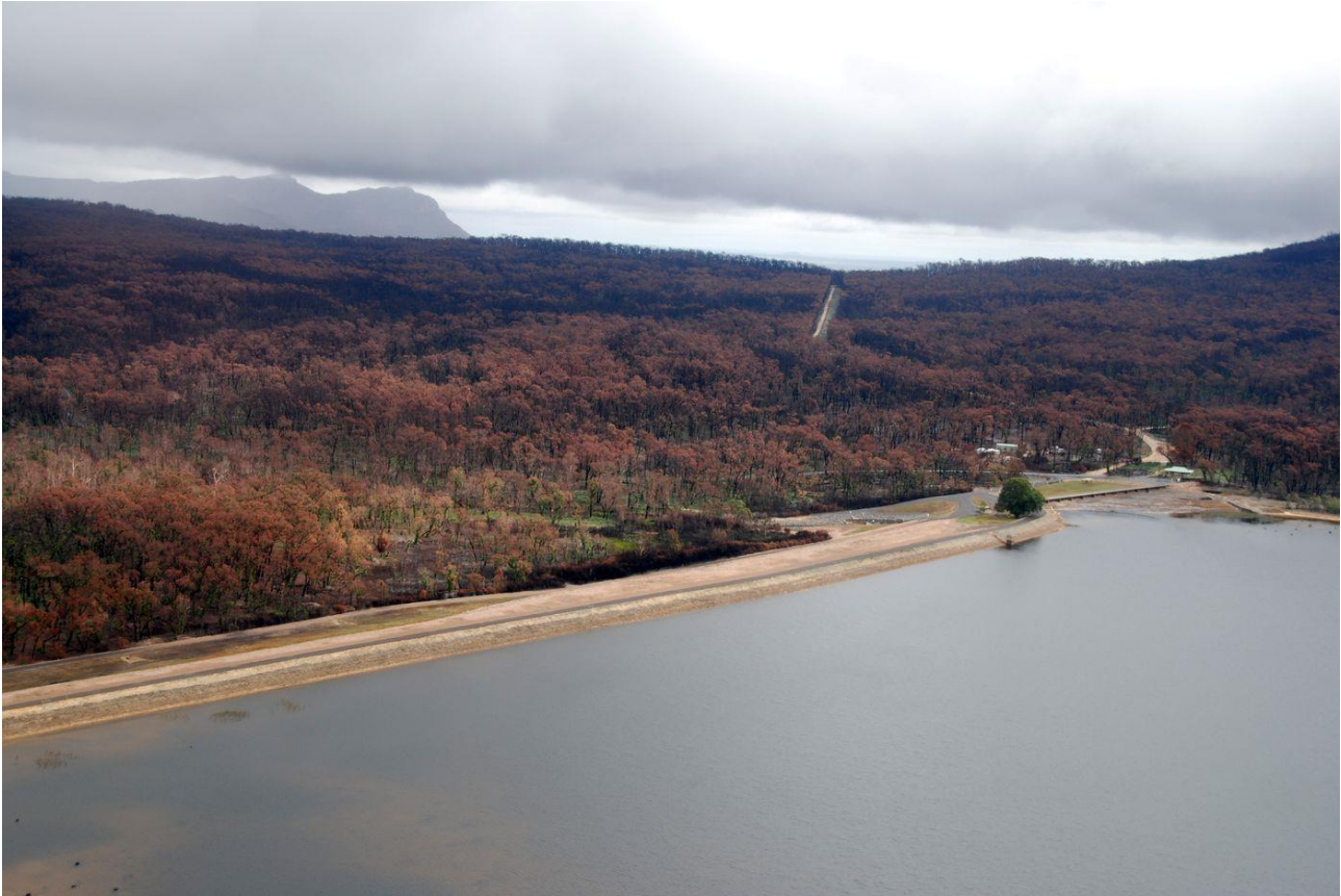
Figure 3-10 Wartook Reservoir – Embankment and spillway (Source: https://www.film.vic.gov.au/choose-victoria/locations/lake-wartook )
