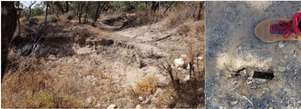
Figure 27. Scour downstream of culvert (left) and tunnelling at Galaquil West Road (right) (YAR078).
