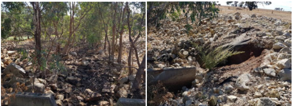
Figure 14. Left: low flow bypass at Jung weir looking downstream, Right: scour of low flow bypass right bank (YAR011)
