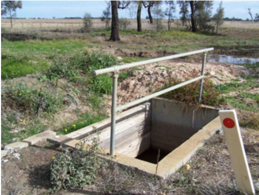
Figure 2-30 Blocked culvert at Lawler Road – Dunmunkle Creek/East Karkarooc Channel
