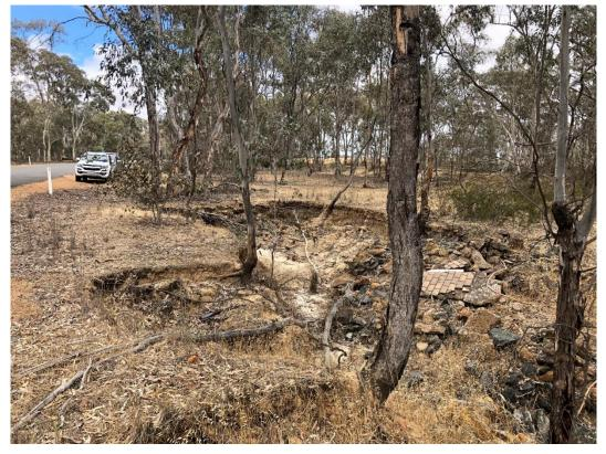
FIGURE 5-10 LOOKING AT THE KNICKPOINT, FORMED THROUGH POOR ROADSIDE DRAINAGE ARRANGEMENTS ENTERING DUNMUNKLE CREEK ON THE CAMPBELLS BRIDGE ROAD.
