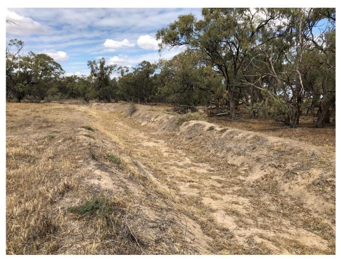
FIGURE 4-5 DOWNSTREAM VIEW OF DUNMUNKLE CREEK, SHOWING A MAN-MADE CHANNEL, UNIFORM BED PROFILE AND SPOIL HEAPS ADJOINING THE CHANNEL, FORMED THROUGH THE PROGRESSIVE CHANNEL ENLARGEMENT WORKS.
