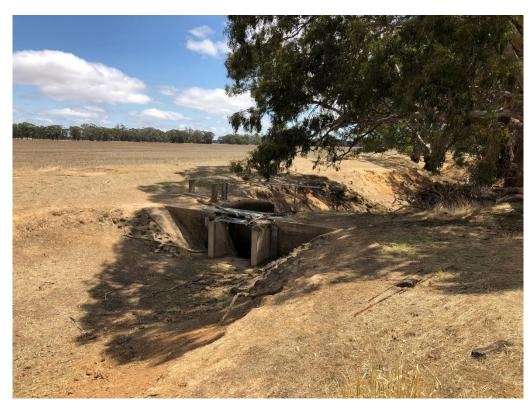
FIGURE 5-18 CONCRETE DROP STRUCTURE IMMEDIATELY UPSTREAM OF THE DUNMUNKLE CREEK-MAIN CENTRAL CHANNEL CONFLUENCE. THE STRUCTURE CONTROLS A CHANGE IN BED ELEVATION.
