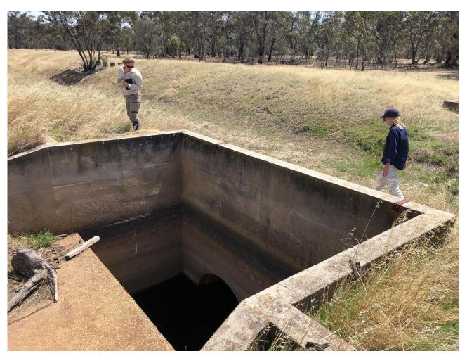
FIGURE 4-8 A SYPHON ON DUNMUNKLE CREEK IMMEDIATELY WHICH FACILITATES FLOW PAST THE ROCKLANDS OUTLET CHANNEL.
