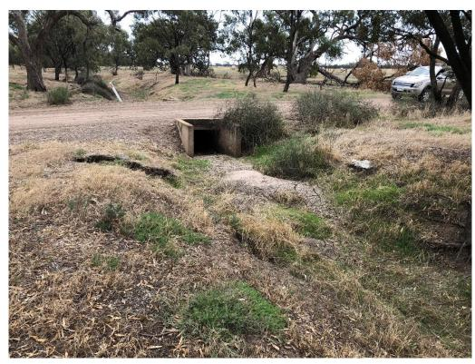
FIGURE 5-31 UPSTREAM VIEW OF THE EROSION AT GORMAN ROAD CROSSING, ASSOCIATED WITH POOR ROADSIDE DRAINAGE ARRANGEMENTS.
