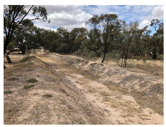
FIGURE 5-27 TYPICAL VIEW OF DUNMUNKLE CREEK SHOWING THE LEVEES ON BOTH SIDES OF THE CHANNEL.
