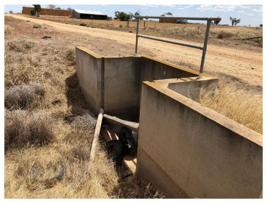
FIGURE 4-6 VIEW OF A REDUNDANT WATERWAY CROSSING OVER A ROAD ON DUNMUNKLE CREEK. THE CROSSING INCORPORATED TIMBER BOARDS TO IMPOUND WATER UPSTREAM.
