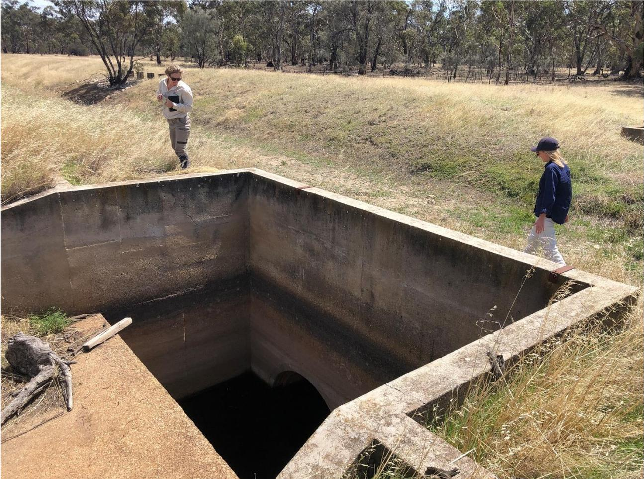
**FIGURE 4-8 A SYPHON ON DUNMUNKLE CREEK IMMEDIATELY WHICH FACILITATES FLOW PAST THE ROCKLANDS OUTLET CHANNEL.**
