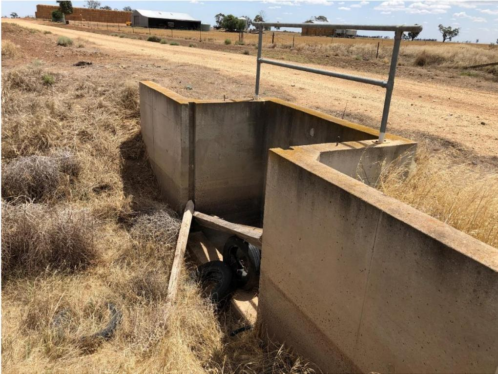
**FIGURE 4-6 VIEW OF A REDUNDANT WATERWAY CROSSING OVER A ROAD ON DUNMUNKLE CREEK. THE CROSSING INCORPORATED TIMBER BOARDS TO IMPOUND WATER UPSTREAM.**
