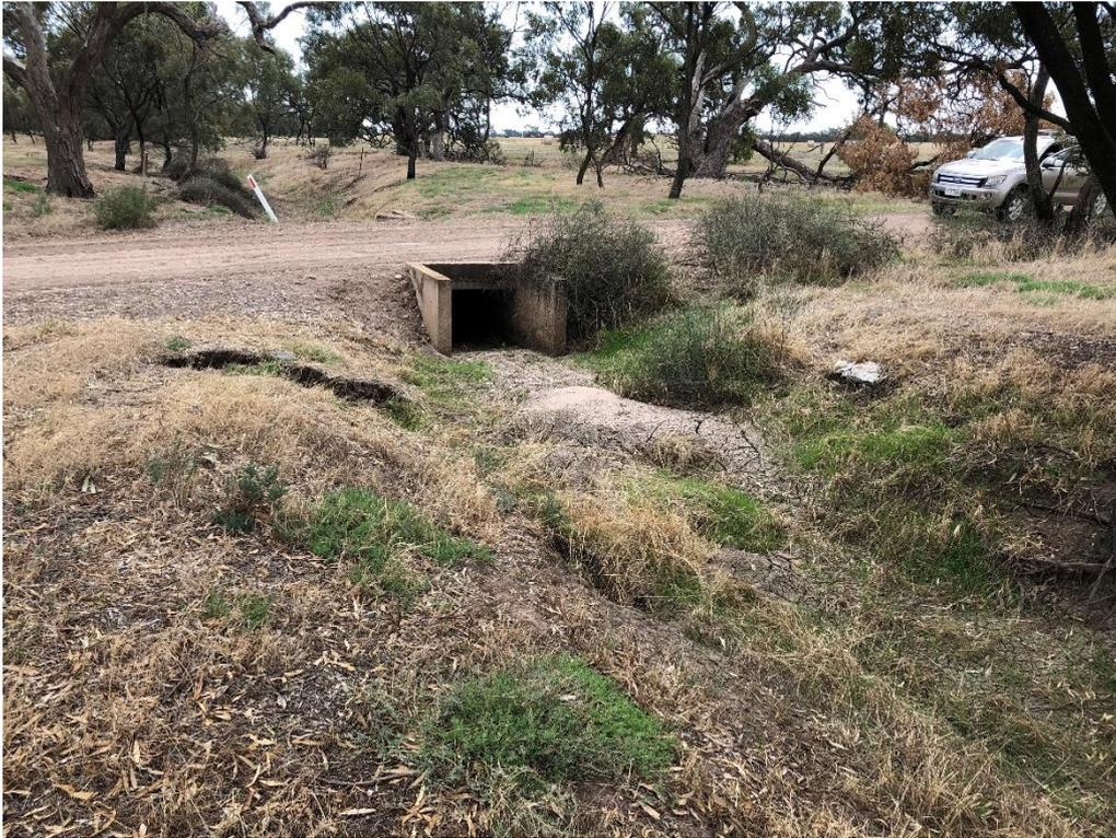
**FIGURE 5-31 UPSTREAM VIEW OF THE EROSION AT GORMAN ROAD CROSSING, ASSOCIATED WITH POOR ROADSIDE DRAINAGE ARRANGEMENTS.**
