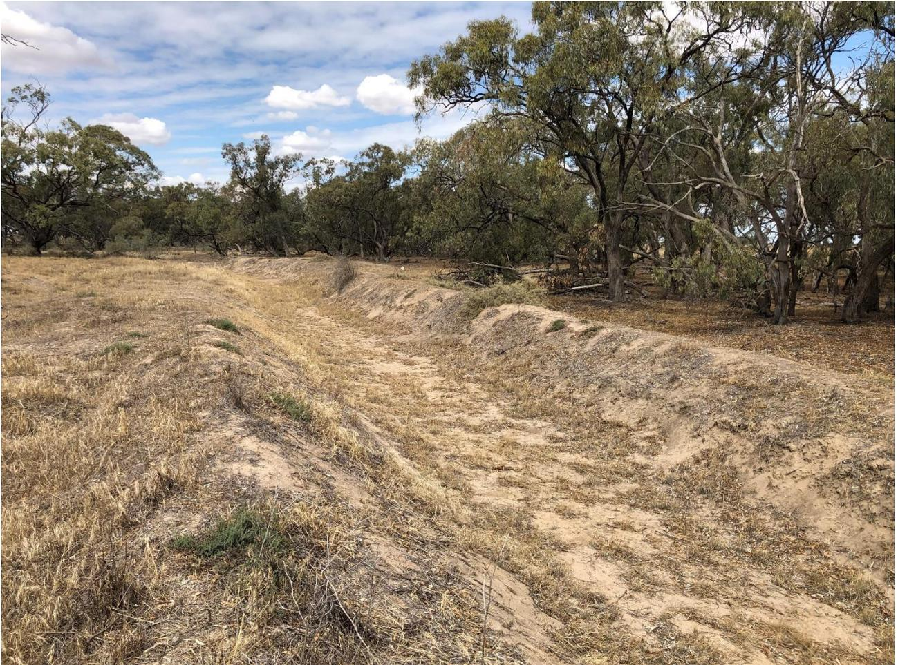
**FIGURE 4-5 DOWNSTREAM VIEW OF DUNMUNKLE CREEK, SHOWING A MAN-MADE CHANNEL, UNIFORM BED PROFILE AND SPOIL HEAPS ADJOINING THE CHANNEL, FORMED THROUGH THE PROGRESSIVE CHANNEL ENLARGEMENT WORKS.**
