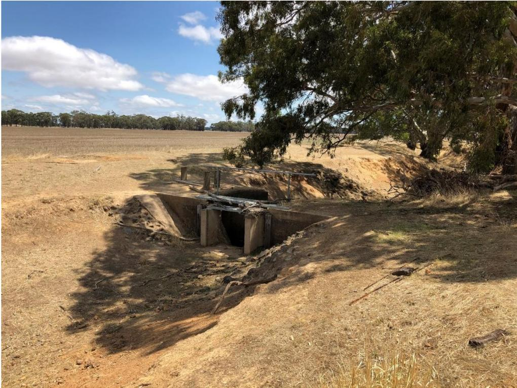
**FIGURE 5-18 CONCRETE DROP STRUCTURE IMMEDIATELY UPSTREAM OF THE DUNMUNKLE CREEK–MAIN CENTRAL CHANNEL CONFLUENCE. THE STRUCTURE CONTROLS A CHANGE IN BED ELEVATION.**
