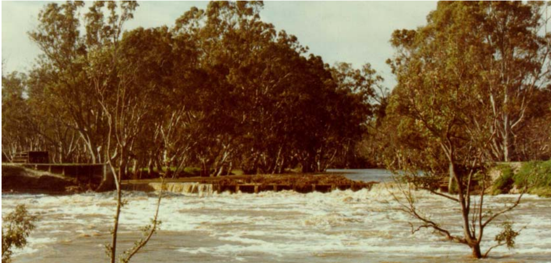
Figure 6.3 Dimboola Weir during the 1981 flood event (1)
