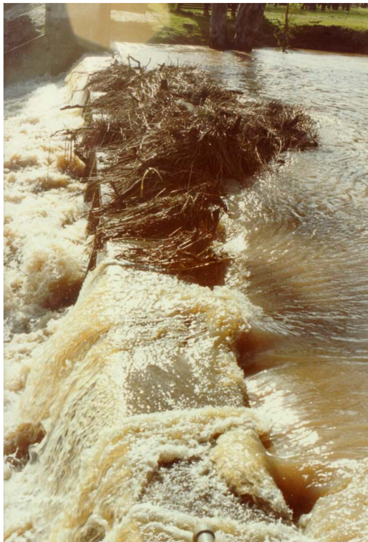
Figure 6.4 Dimboola Weir during the 1981 flood event (2)
