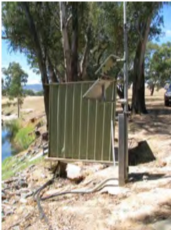
Figure 3-3 Wimmera River at Eversley Stream Gauge
