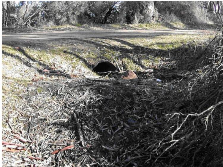
**Figure 10. Peuckers Rd crossing of Burnt Creeks showing the bank constructed on the upstream side**
