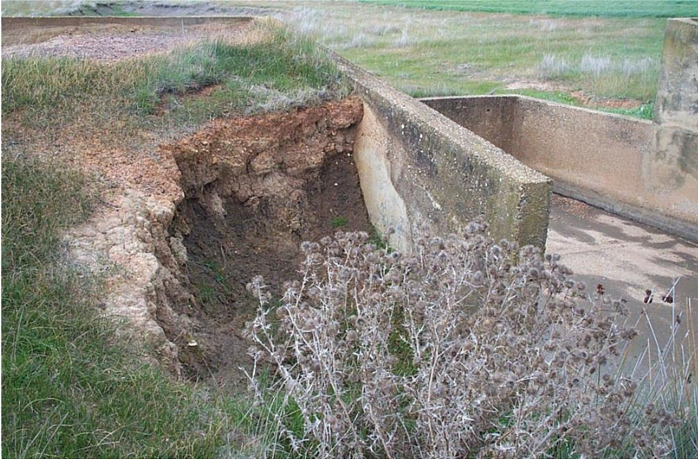
*Figure 7. Scour hole on the right bank of the downstream end of the smaller Astons Scour drop structure. The missing wing would have been attached to the end of the concrete wall beside the scour hole.*
