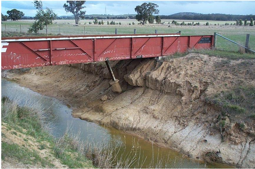
Figure 11. Soil loss around the supports of a private bridge crossing Six Mile Creek
