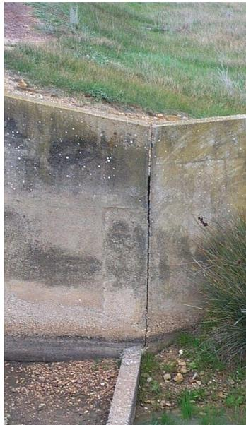
*Figure 8. Crack in the left bank downstream end of the smaller drop structure on Astons Scour.*
