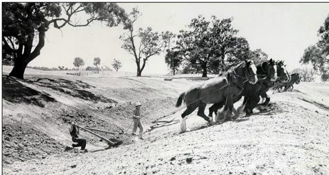
Figure 2 Constructing the open channels in the Wimmera. Photo supplied by GMMWater
