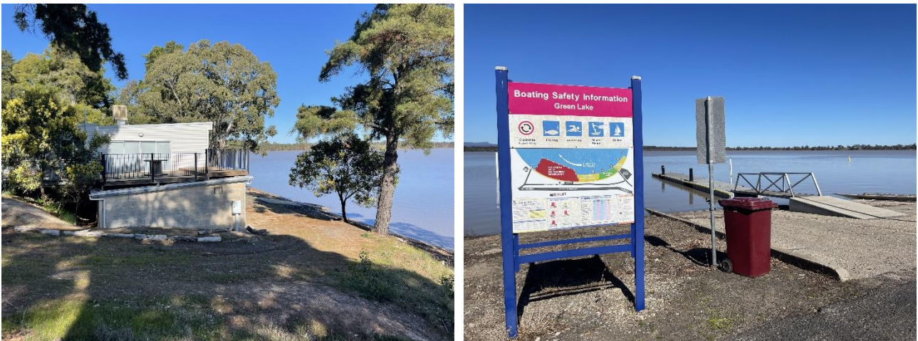
Figure 5-4 Foreshore infrastructure includes the Yacht Club (left) and the main boat ramp (right)
