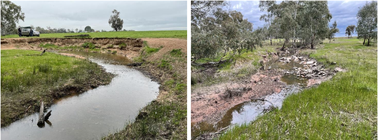
Figure 5-12 Erosion sites including a deepening meander cutoff (left), and outside bend migration (right)
