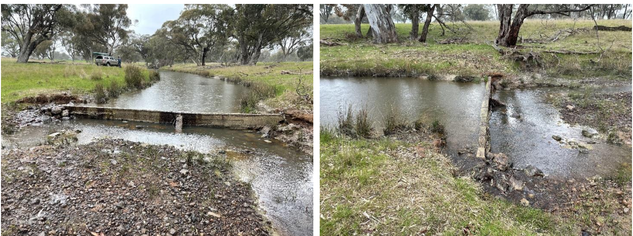
Figure 5-13 Small weir and weir pool
