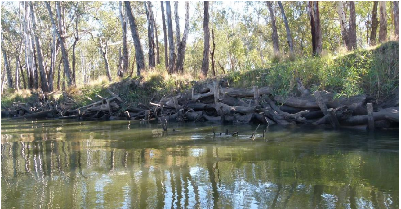
Figure 7-2 Log revetment on the Murray River (sourced from Soil Conservation Service).
