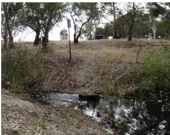
Figure 4-19: Concrete sill on the Wimmera River (left) and Yarriambiack Creek (right) that split all but flood flows between the two waterways.
