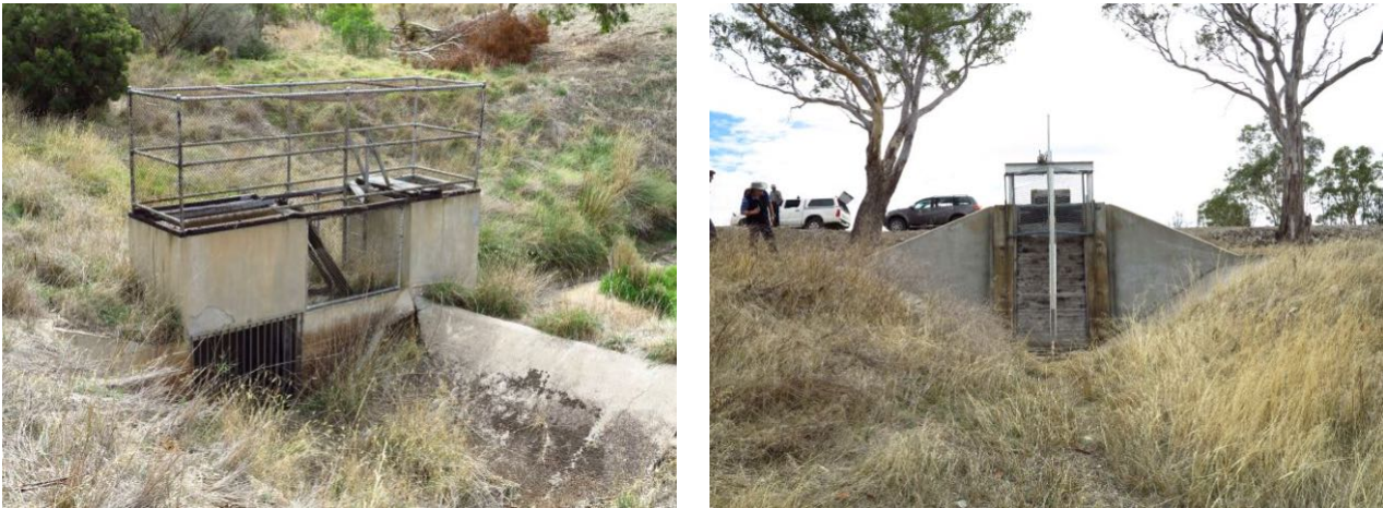
Figure 4-16: Regulator structure at the inflow pipe from Green Lake to Dock Lake (left) and regulator on the outfall channel from Dock Lake to Burnt Creek (right) (Source: Jacobs, 2015)
