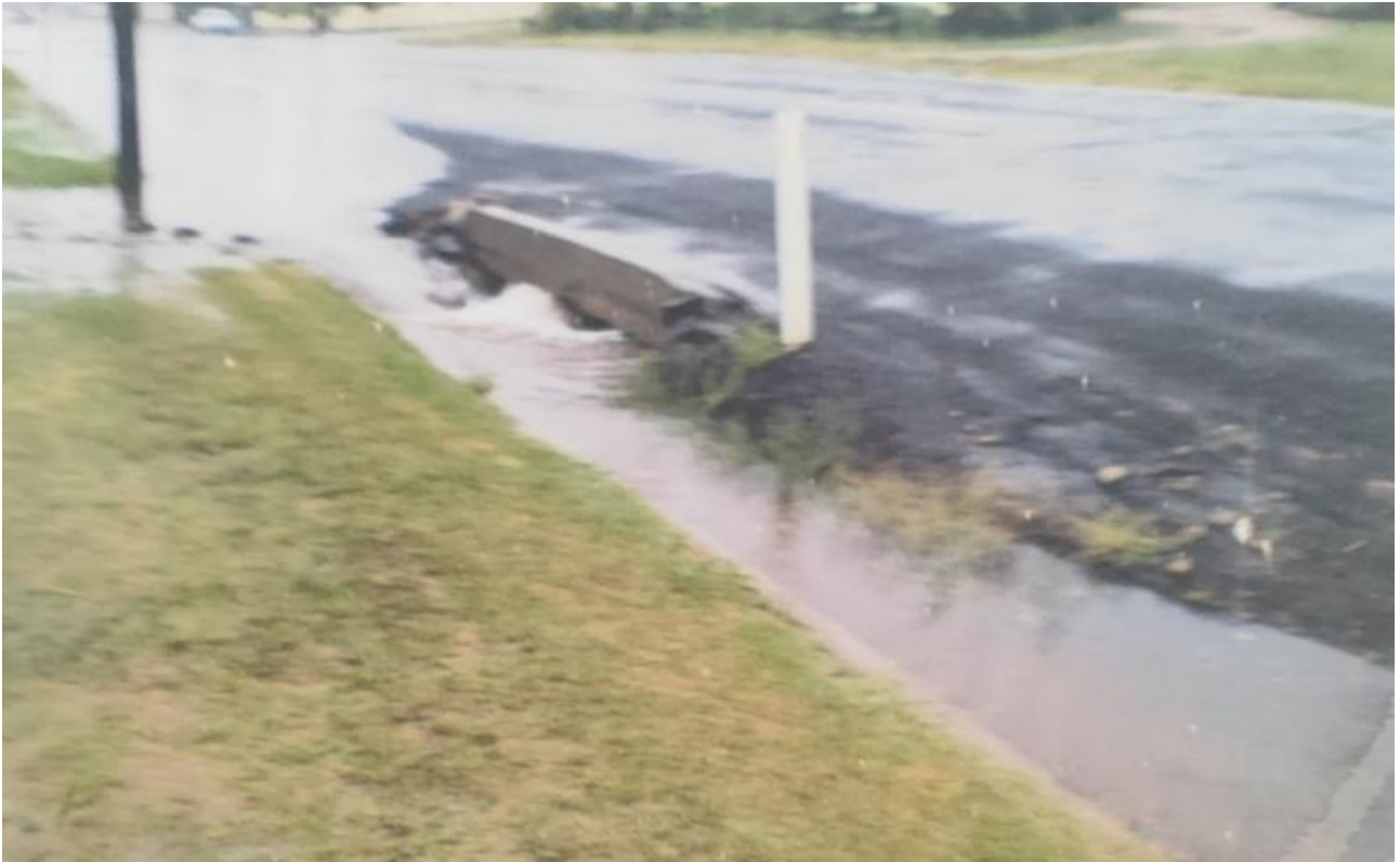
Figure 2-7 Flooding at Wallace Street Crossing
