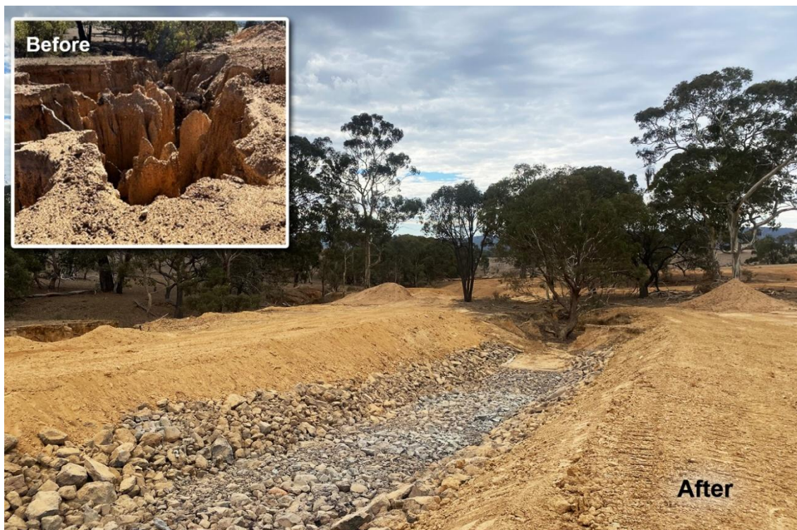
Works underway in an upper catchment waterway to reduce sediment movement and impacts downstream.
